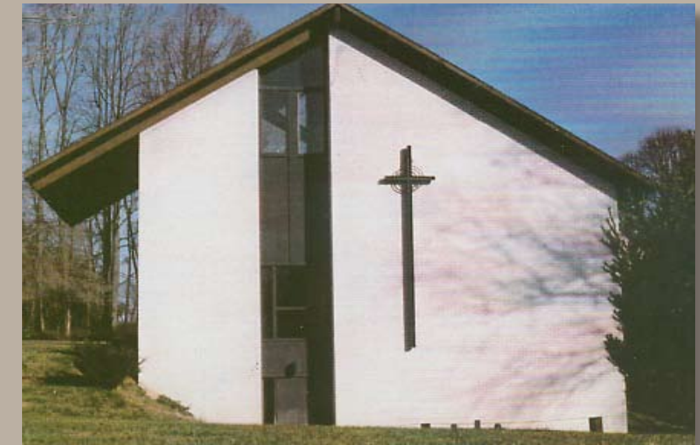
Above: Original Christian Education Building, dedicated June 1967
